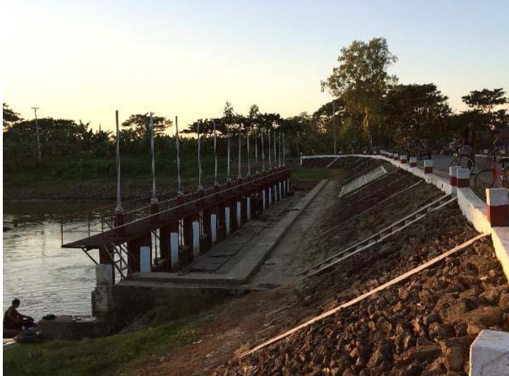
Water control infrastructure, Maubin township
